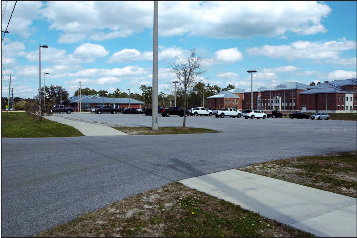
PLATE 6: Looking Northeast at BEQ (RR122) and EM Dining Facility (RR135), Stone Bay Rifle Range Historic District, Camp Lejeune, North Carolina
