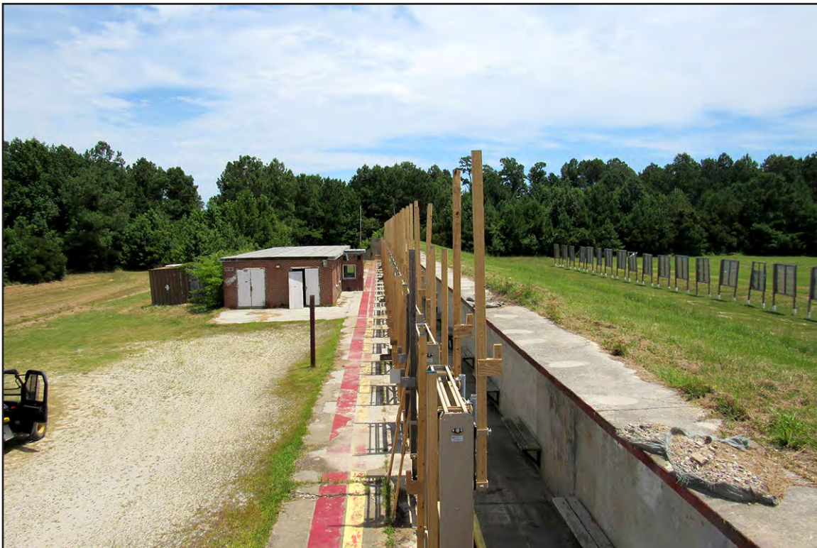
PLATE 2: Range Bravo, Looking East, Showing Concrete Wall and Butts, Stone Bay Rifle Range Historic District, Camp Lejeune, North Carolina
