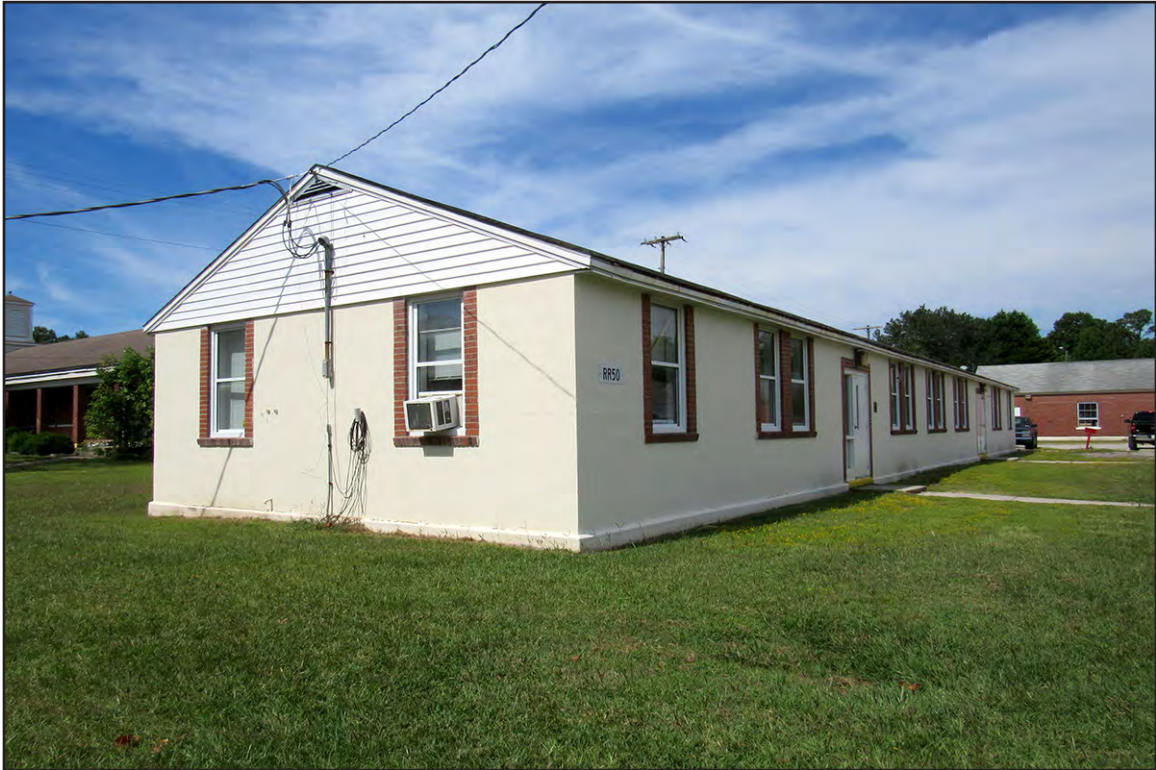
PLATE 22: RR50, East and North Elevations, Stone Bay Rifle Range Historic District, Camp Lejeune, North Carolina
