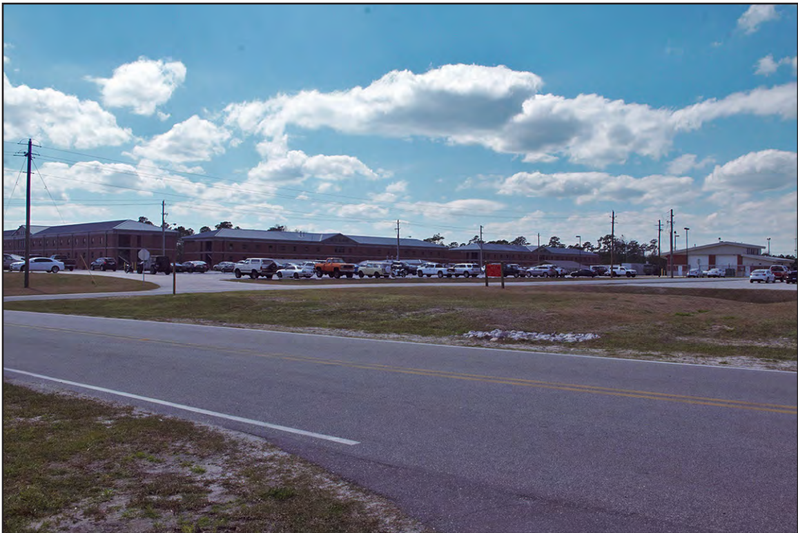
PLATE 7: Looking Southwest Across Range Road at the Southern End of the Stone Bay Rifle Range Historic District, Camp Lejeune, North Carolina
