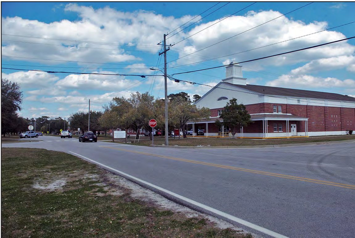
PLATE 12: Theatre/Gymnasium Combination Building (RR8), Oblique of West and South Elevations, Looking Northeast on Range Road, Stone Bay Rifle Range Historic District, Camp Lejeune, North Carolina
