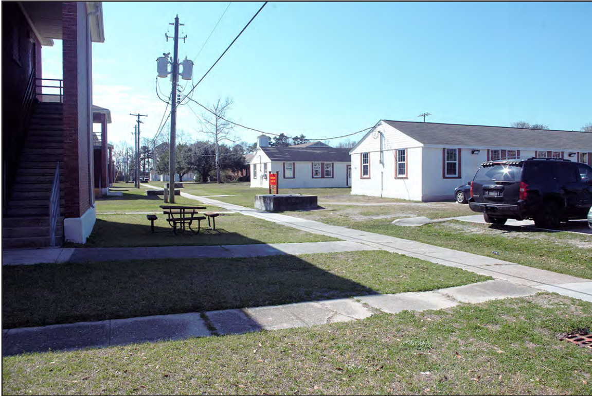
PLATE 11: Looking South Toward Barracks Buildings and RR51, Stone Bay Rifle Range Historic District, Camp Lejeune, North Carolina (Hardlines 2006)
