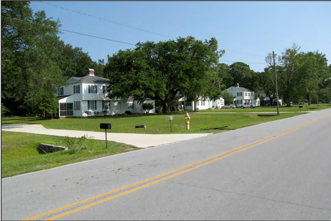
PLATE 24: Range Road, Looking Southeast Toward Former Family Officers' Quarters (now demolished), Stone Bay Rifle Range Historic District, Camp Lejeune, North Carolina (Hardlines 2006)
